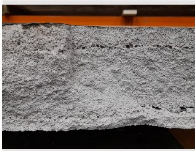
Photo showing bubble formation on reinforcement
